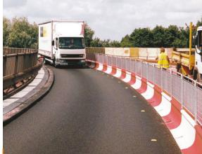
**Barrier Specifications** Length: 1.5m Height: 0.42m Base Width: 0.50m Weight: 48kg
